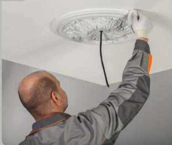
Wipe the area of the junction with a wet cloth. Wet the cloth with water if G06M290 Adhesive is used and with Acetone in case of using G08S60 / G07S290.
