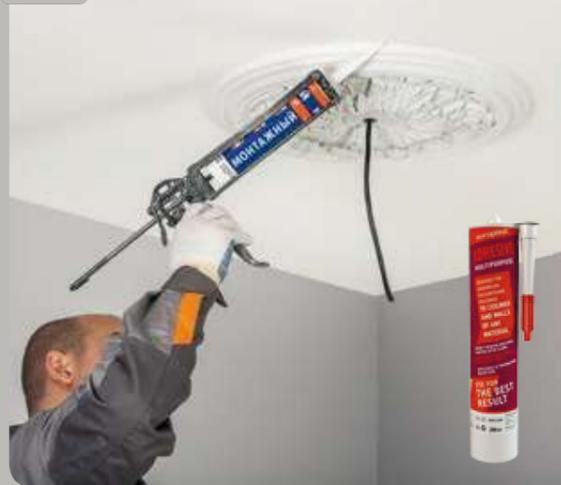
Fill the spaces in the junction area between the cornice and the walls/ ceiling, where the adhesive has not shown on a surface.
